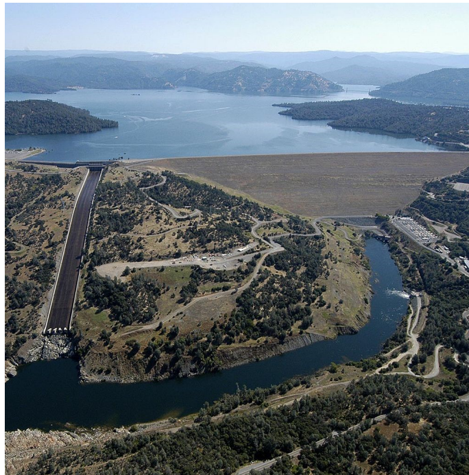
View of Oroville Dam and Lake Oroville in background, in 2005.
